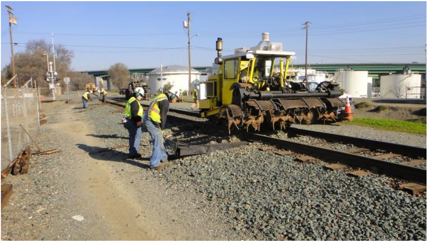
Alan operates the scarifer's inserter function to install new ties while Heather and Steve guide it into place.
