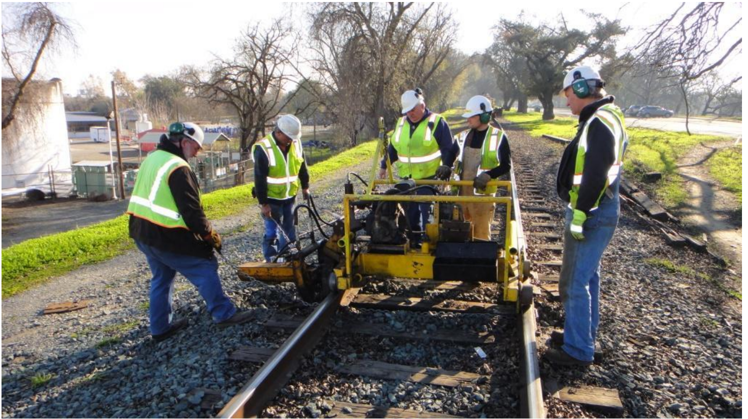
In the afternoon, more bad ties are pulled. Frank and John adjust the chains. DJ operates the section-gang machine while Harry and Steve take in all the action...
