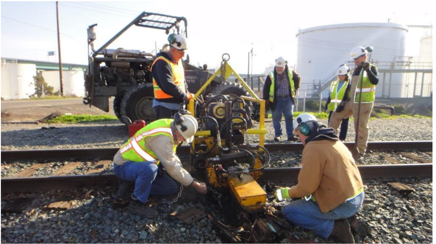
This rotten tie just disintegrated under the hydraulic power of the section-gang machine. So, we implemented the chain method of pulling the tie out from behind. Alan and Steve adjust the chains as Fred operates the machine.
