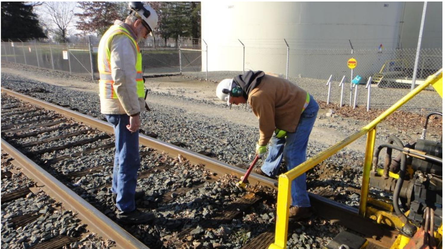
Alan supervises as Steve uses the adze to shave off the top of the tie that was binding on the base of the rail.
