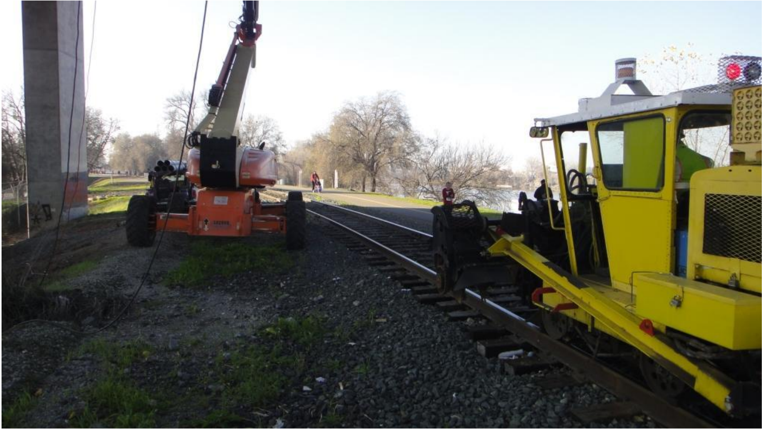
It's a stand-off! Fortunately the MOW Team was able to give this CalTrans crew a refresher in Part 214...
